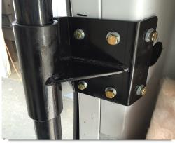
4) Install the (2) 5/16" rivet nuts into the 1/2" holes. Using the rivet nut installation tool tighten down the rivet nut securely. Refer to photo below.
